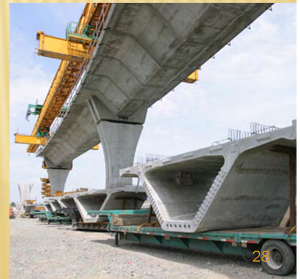
Concrete Segmented Bridge
